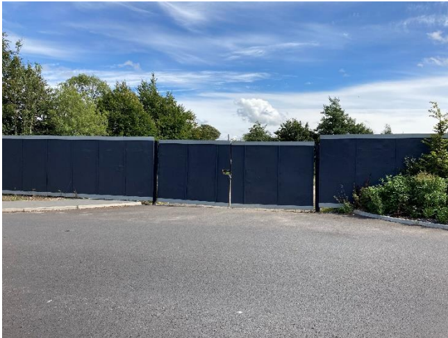
Photograph 1: Existing Site Access
