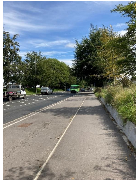
Photograph 9: Pedestrian footway along Christy's Lane
