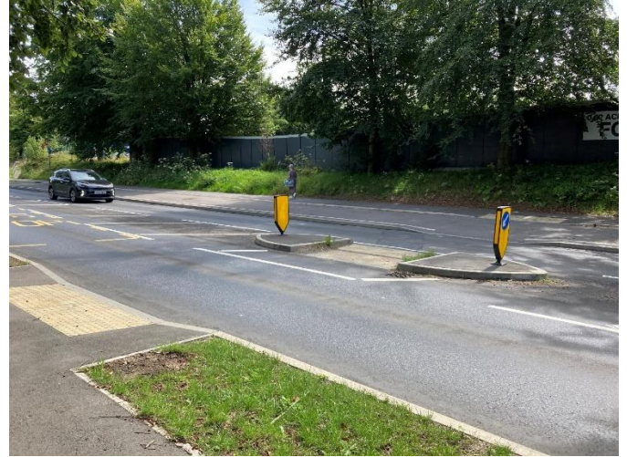
Photograph 6: Pedestrian crossing point present over Christy's Lane
