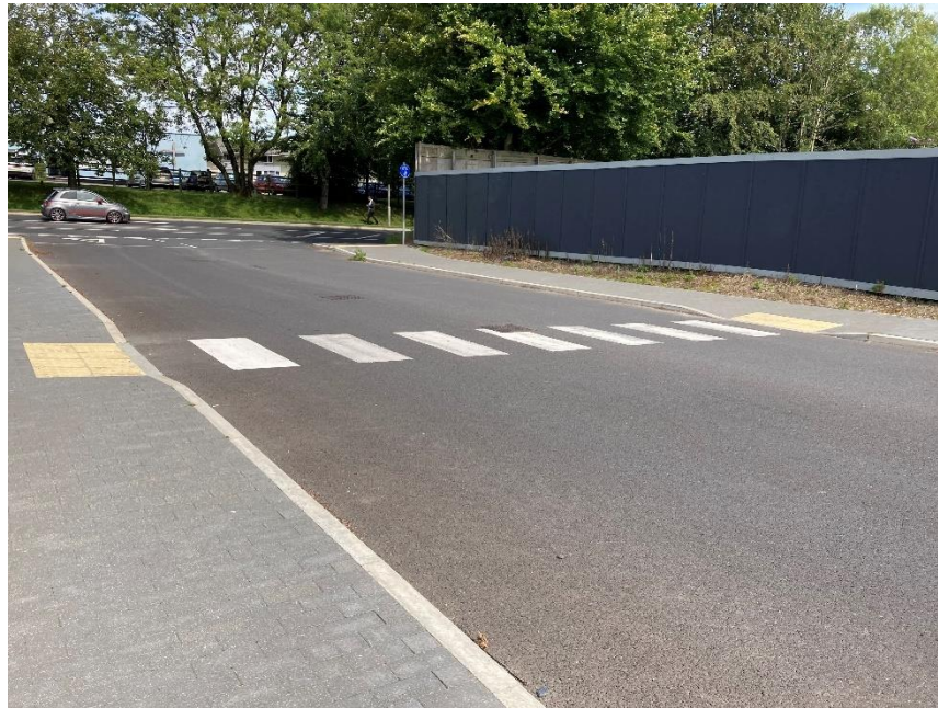
Photograph 7: Pedestrian crossing point adjacent to the site
