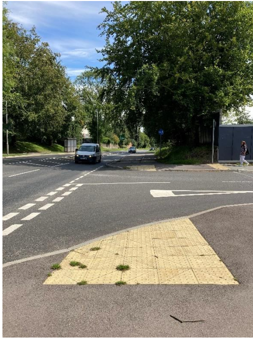
Photograph 8: Tactile paving present at the access
